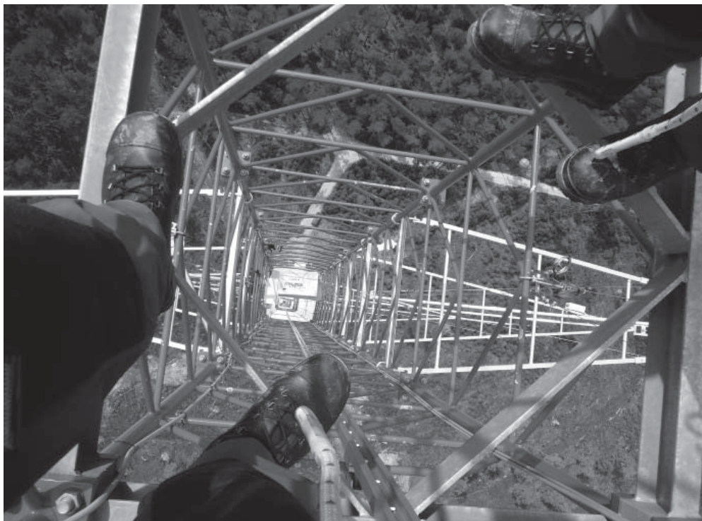
Specialists install the 200-meter high measuring mast.
