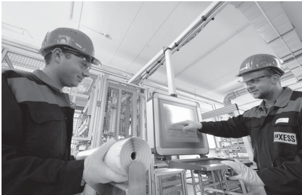
The membrane elements for water treatment are manufactured in the semi-automatic system in Bitterfeld. A single membrane element consists of a bundle of over 20 layers. It is aligned with a winding module and secured. The LANXESS employee (left) is holding such a module. (© LANXESS AG) | Picture in color and printing quality: www.fraunhofer.de/press
