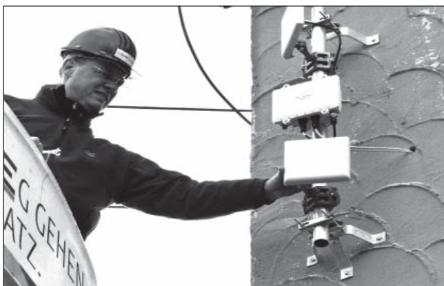
A researcher positions a WiBACK network antenna. (© Fraunhofer FOKUS)
