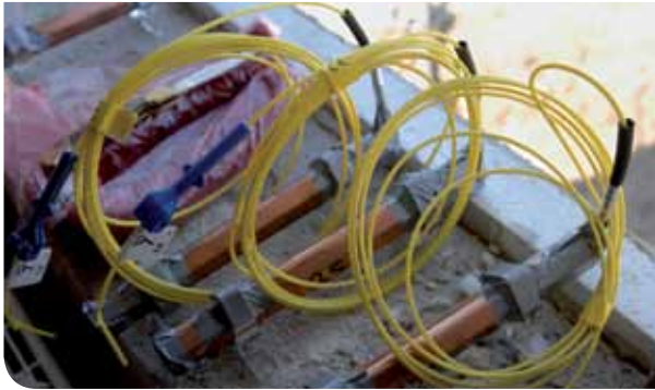
Specially-prepared cutting charges for cutting the steel girders in the building's interior.
