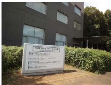
The front of the building.
