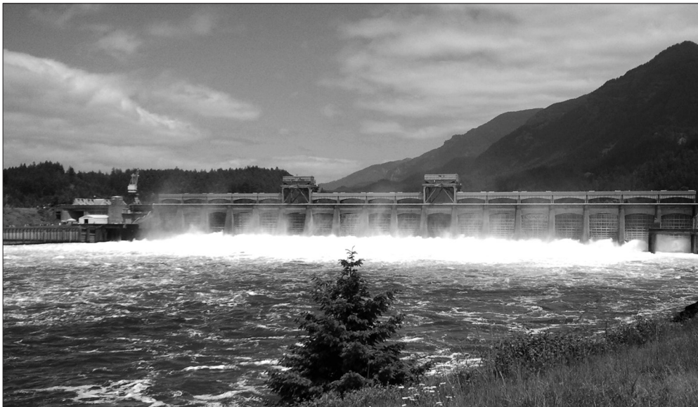
The hydroelectric plants in the Columbia River basin in the Pacific Northwest generate 22,000 MW in output. In the photo: a dam wall in the many-branched dam system. (© Fraunhofer IOSB) | Picture in color and printing quality: www.fraunhofer.de/press
