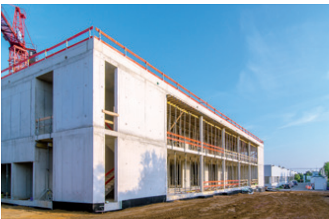
View of the construction site (facing east)
